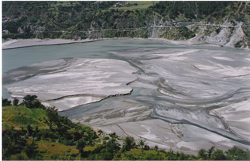
Picture 1: Problem of Siltation in Chamera Dam
