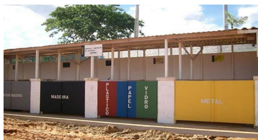
Fig.4: Wooden bins for the collection of construction waste
