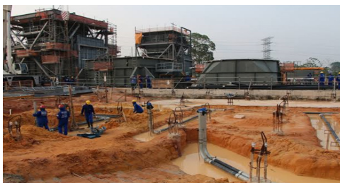
Fig.2: Construction Site of a Thermoelectric Plant
