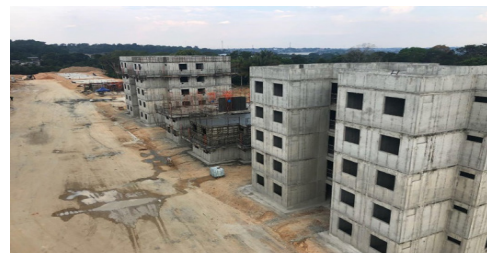
Fig.3: Construction site for residential buildings
