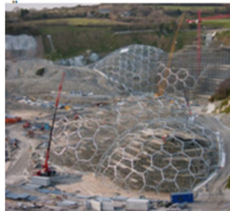
Fig. 18: Working equipment in the site
