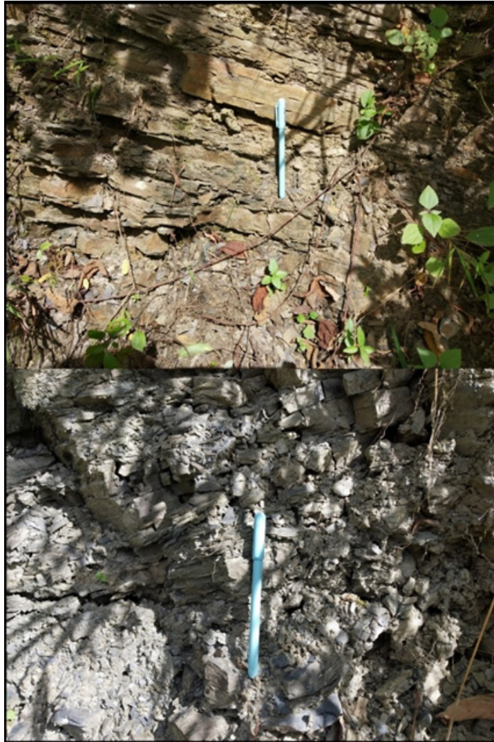
Fig. 2: Rock exposures showing fractured and weathered shales.
