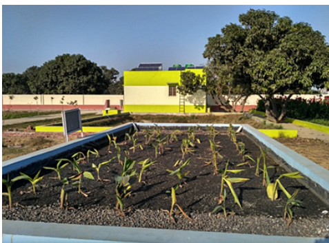
(c) Start-up Phase of the bed of HSSF CW
